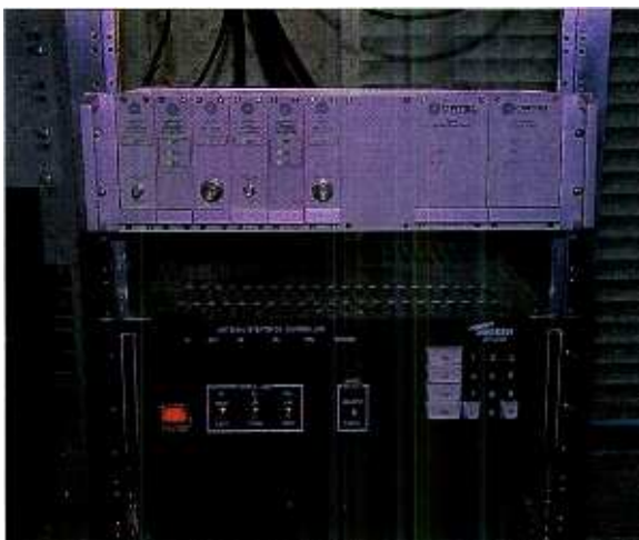
This rack at a station's remote downlink contains fiber-optic terminal equipment (above) and satellite antenna controller (below). (Courtesy of WBBM-TV, Chicago.)
